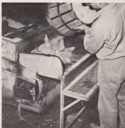
FIGURE 1.—A basket of sweetpotatoes is dumped on a chute of iron rods. Loose soil falls through the rods but the sweetpotatoes usually receive some injuries.
